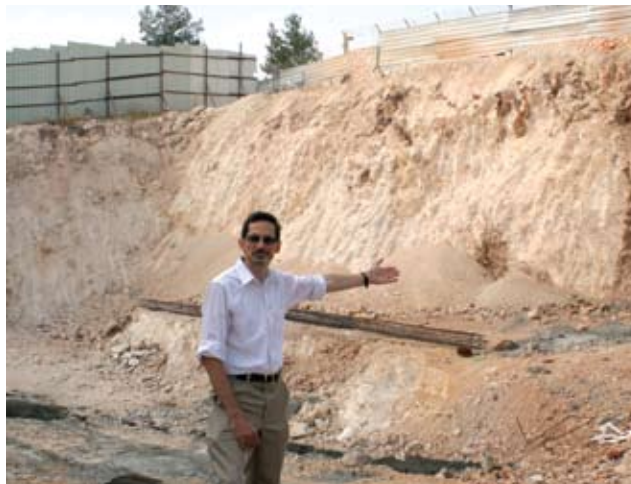
Prof. David Golinkin inspects campus excavation work
